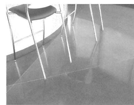
Lobby, corridor and break-room floors in the EOC and Logistics Buildings are polished, stained concrete similar to those in this photo of the Wiginton Hooker Jeffry office. This was a less costly, durable and resource-conserving alternative to porcelain tile or other hard-surface floor coverings.
